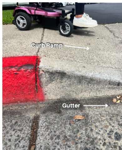
Figure 1. This image depicts the curb ramp and gutter of a sidewalk. The PWC might shift towards the gutter unless speed is adjusted and joystick is appropriately used.
